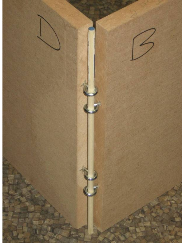
Figure 44: Dowel Joining Two Walls
